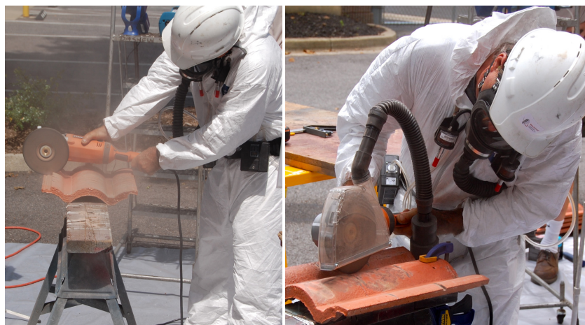
Figure 6.2. CPWR demonstrates the effectiveness of ventilation with construction nanomaterials. Here, a worker using a tile cutter on a clay roofing tile and producing a large amount of clay dust (on the left) can control exposure using a fitted vacuum hood (on the right). (Images courtesy of B. Lippy.)
